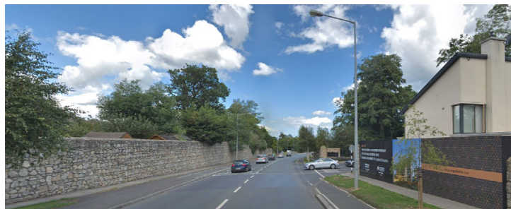
View 1 - from North down Brewery Road
