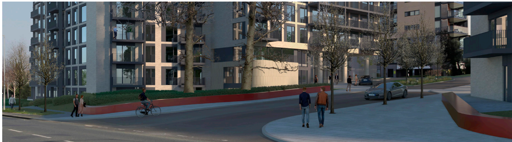
Block H's lower levels as seen from the site's entrance
